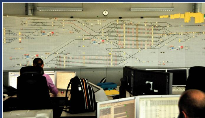
This is the control room at Zürich-Limmattal marshalling yard, the „heart“ of the „hub-and-spoke“ system. Here wagonload freights are handled three times daily, involving the remarshalling of over 2,500 wagons.
